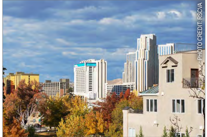
Example: Varied building heights and forms
