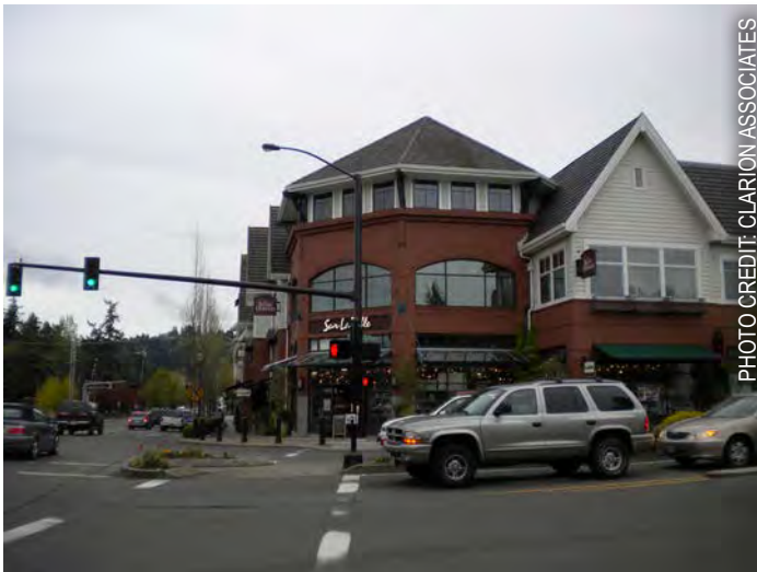
Example: Mixed-used building in a neighborhood setting (Lake Oswego, OR)
